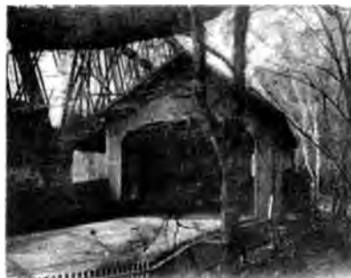
WEST RIVER BRIDGE
